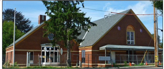
(current picture of library under construction)
